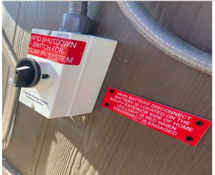
Battery E-Stop examples. Plus the extra required placard. A padlock must fit through the locking mechanism.
