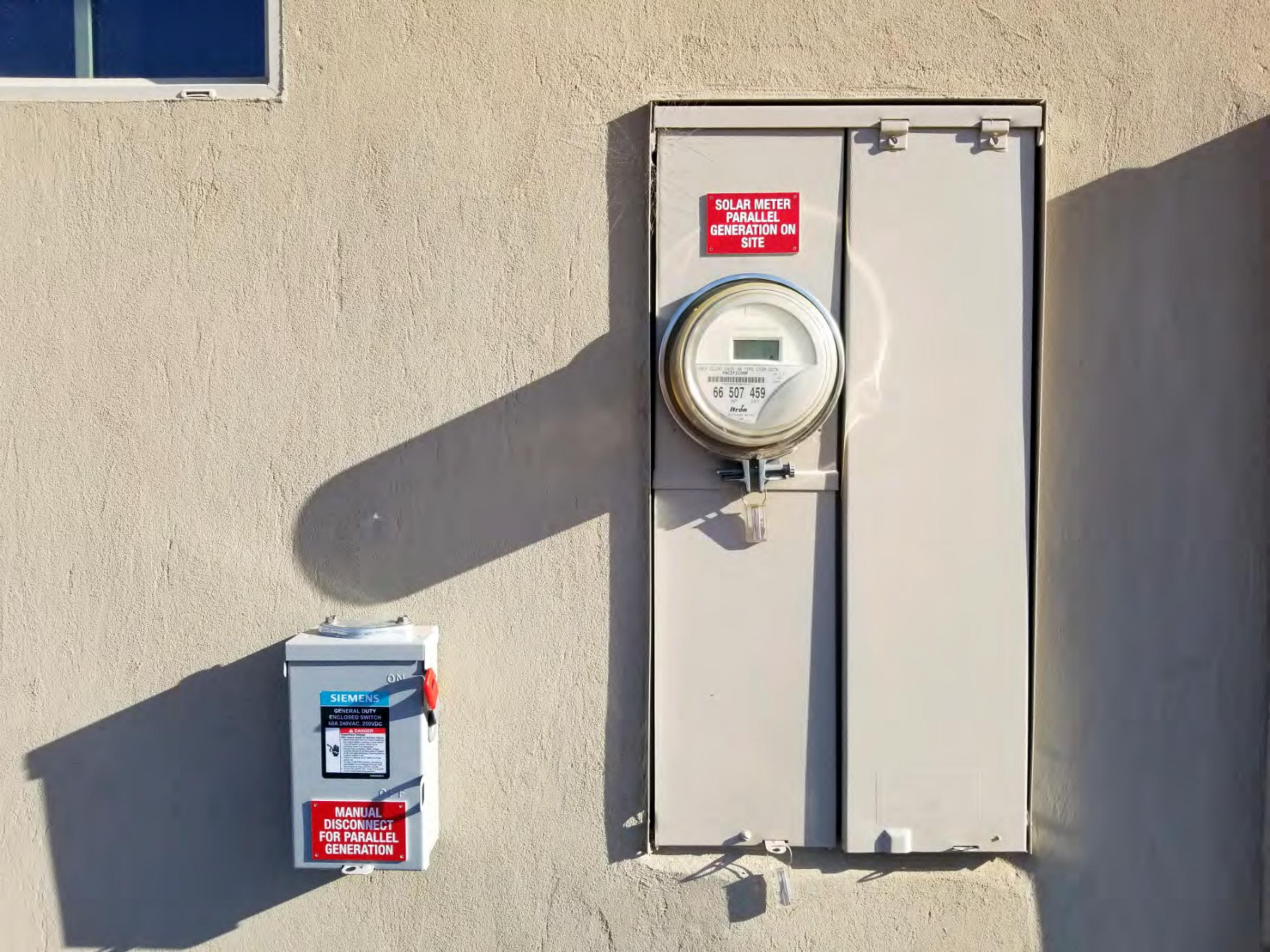
DC Coupled: The solar and battery share the same inverter ALWAYS one knife blade type AC disconnect for both. Labeled with both the ac disconnect engraved label and the battery disconnect engraved label.
