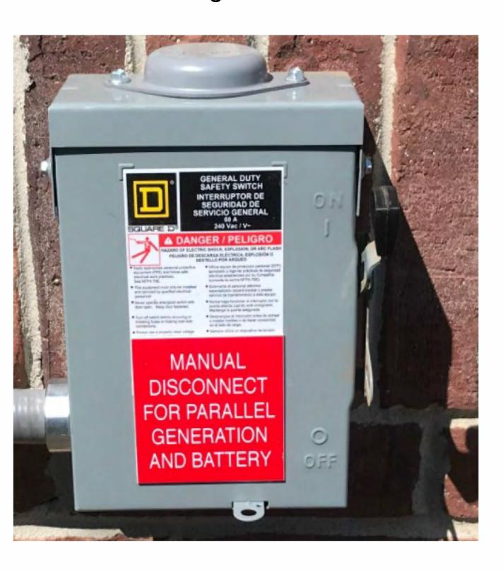
This is an example of using an E-stop button (or other switch) that can shut off the battery system.
