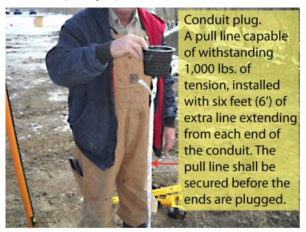
Figure 26—Conduit Plug and Pull Line
