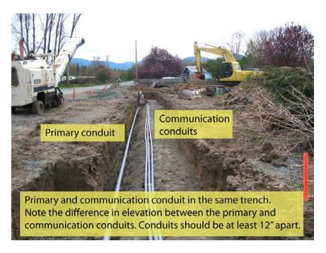
Figure 8—Power and Communication Conduits in Trench
