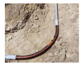
Figure I 6—Field-Installed Elbow
