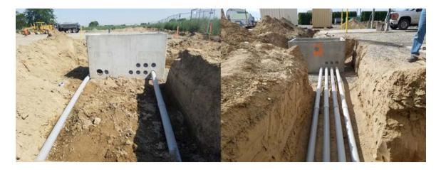
Figure 20—Typical Conduits Attached to a Padvault and Communication Conduit
