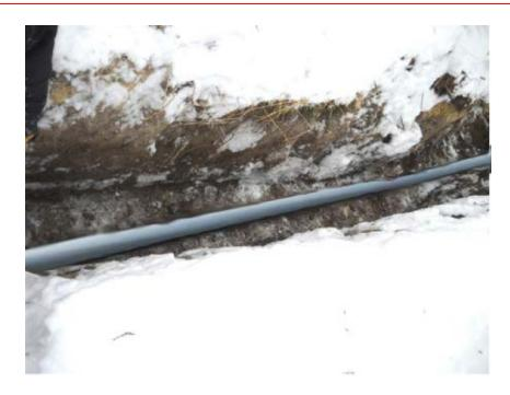
Figure 5—Typical Conduit Trench
