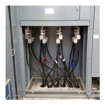
Figure 40—Example of Correct Conduit Installation
