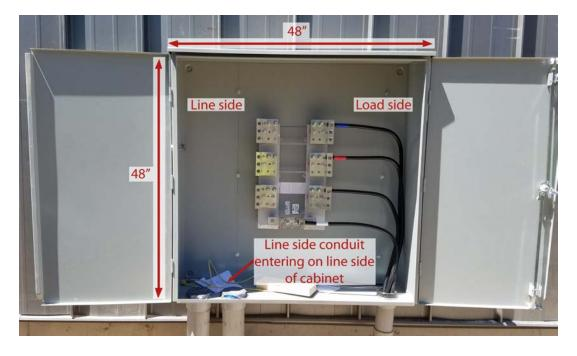
Figure 38—Example of Correct Cable Pulling into Bottom-Entry Line and Load CT Cabinet
