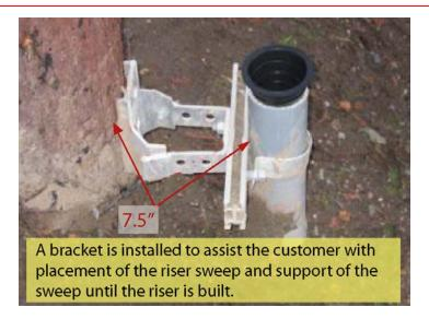
Figure 30—Riser 7.5" from Pole, Bracket
