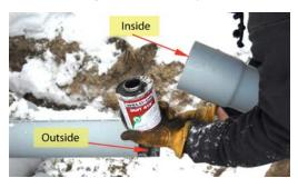
Figure 24—Applying Glue to Conduit
