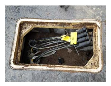
Figure 65—Example of Proper Conduit Installation for Flat Lid Top
