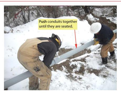
Figure 25—Seating the Conduit
