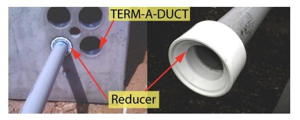
Figure 21—Reducer Used for Conduit Entering the Padvault
