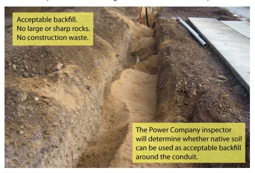
Figure 12—Acceptable Backfill
