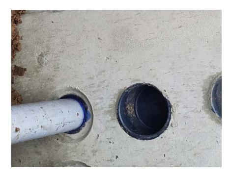
Figure 22—Proper Installation of Conduit into Term-A-Duct
