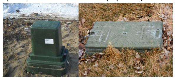
Figure 58—Above Grade Pedestal and Flat Lid Installed on Secondary Boxes
