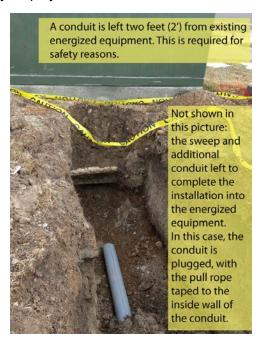
Figure 19—Installing Conduit to Existing (Energized) Equipment
