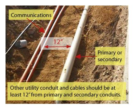
Figure 10—Joint Trench for Primary/Secondary with Communication
