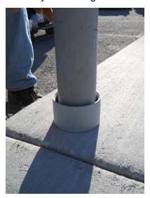
Figure 23—Installing Conduit through Concrete
