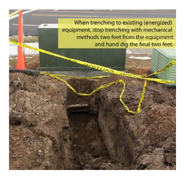
Figure 3—Trench to Energized Equipment
