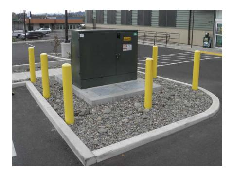
Figure 46-Barrier Posts, Example
