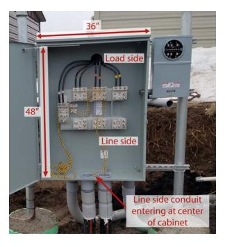
Figure 36—Example of Correct Cable Pulling into Top-Half Load CT Cabinet
