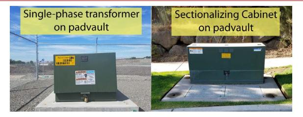
Figure 48—Examples of Transformer and Sectionalizing Cabinet on Padvaults
