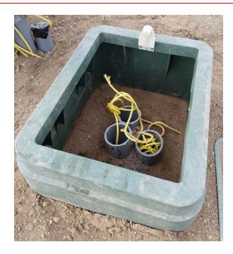
Figure 64—Example of Proper Conduit Installation for Pedestal Top
