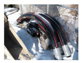
Figure 15—Fiberglass Sweeps with PVC Ends
