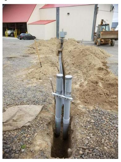
Figure 29—Riser When No Pole is in Place
