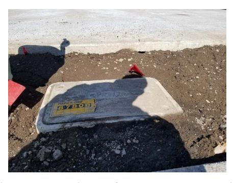
Figure 61—Installed Fibercrete Secondary Box Base and Flat Lid
