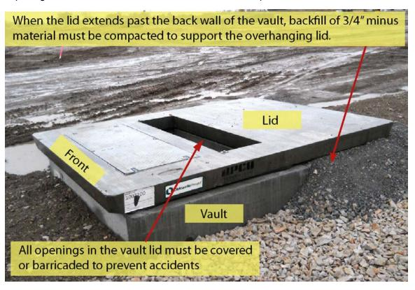
Figure 47—Correctly Installed Padvault in Non-Pedestrian Area
