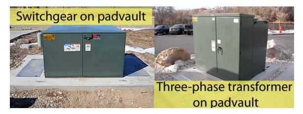
Figure 49—Switchgear and Three-Phase Transformer on a Padvault
